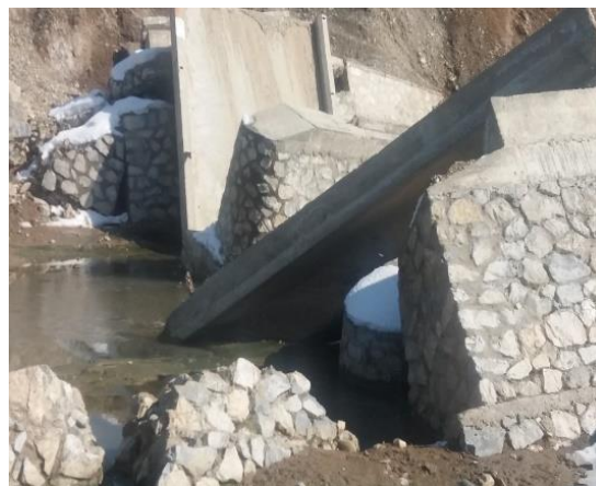
Photo 4-57: Chamni village: damaged culvert
