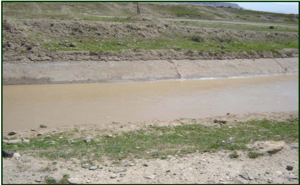
An irrigation channel in Balkh (Third Dekad of March 2006)
